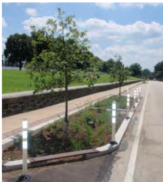
FIGURE 9: Stormwater “Bumpout”, Queens Lane, Philadelphia.
