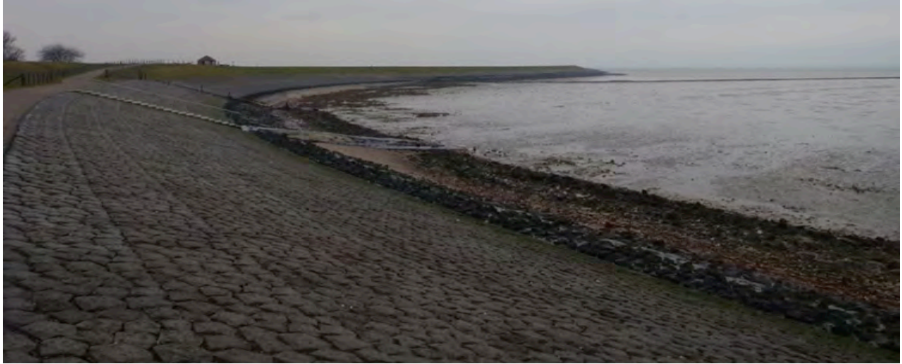
FIGURE 5: Armored levee in the Netherlands at low tide (Cornell et al., n.d.).
