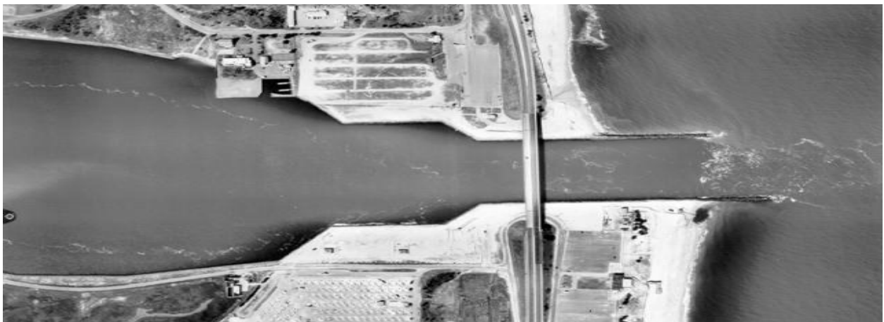
FIGURE 9: Jetties at Indian River Inlet, DE with updrift accretion and downdrift erosion (Cornell et al., n.d.).
