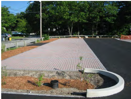
FIGURE 12: Pervious pavers, pervious asphalt and a bioretention cell in Wilmington, MA (GeoSyntech).
