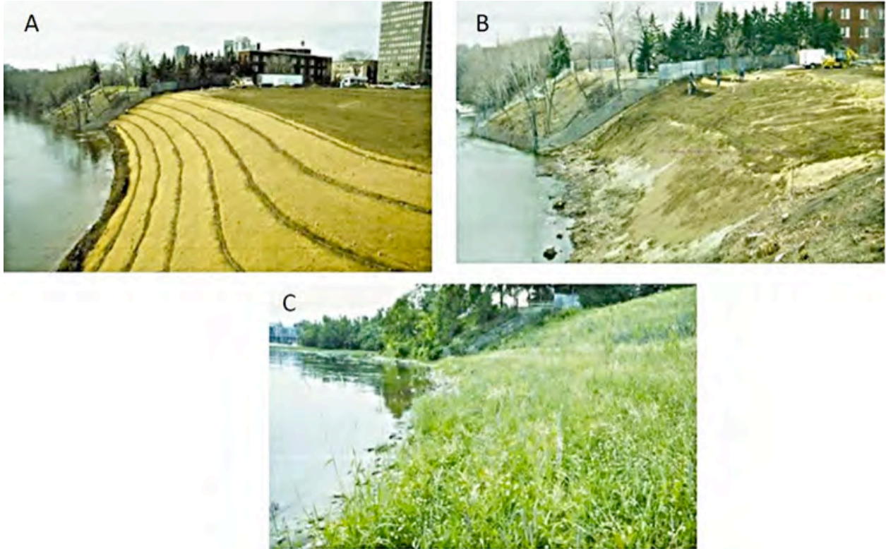
FIGURE 12: Phases of streambank stabilization (A) excavation of undesirable material, (B) new topsoil added, and (C) the final product with stream banks overgrown with lush vegetation (Cornell et al., n.d.).
