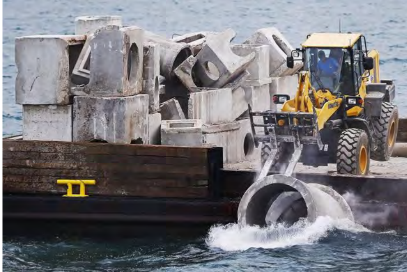
FIGURE 5: Photographs of concrete being dropped in the Gulf of Mexico off of Marco Island, Florida for the creation of artificial reef habitats (Naples Daily News, Jan. 2015).
