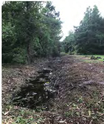
After Prep Work June 14
