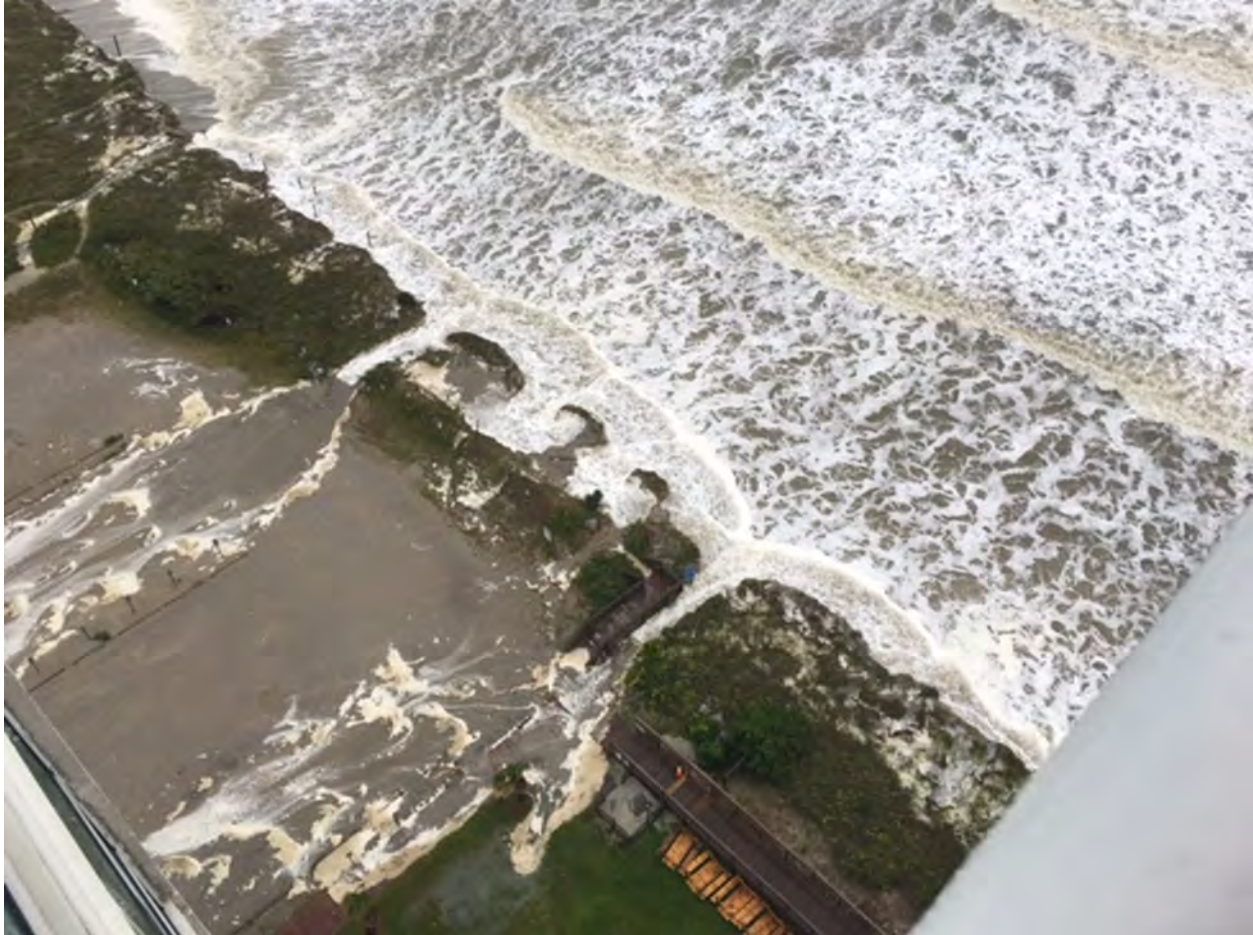
FIGURE 2: Photograph taken from a high-rise hotel in North Myrtle Beach looking down on the beach/dune system during the passage of Hurricane Matthew in October 2016. Note the storm surge pouring into the public infrastructure by way of the low areas between the dunes.
