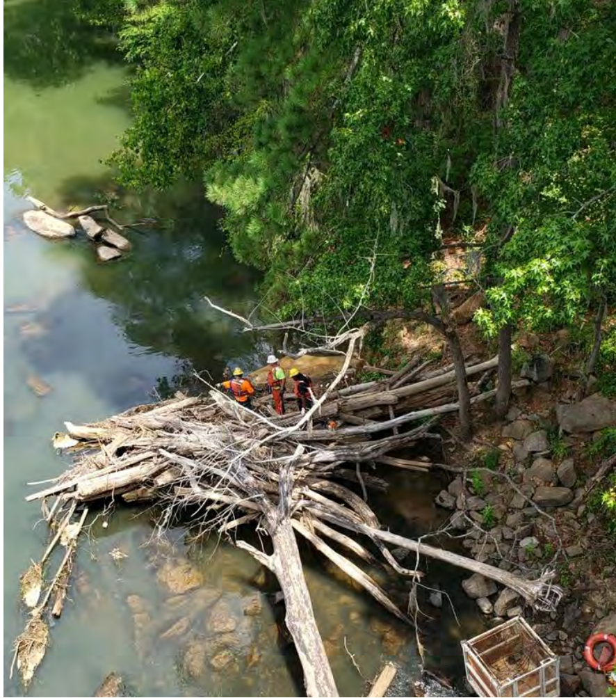
FIGURE 3: SCDOT clearing accumulating debris adjacent to a major bridge structure.
